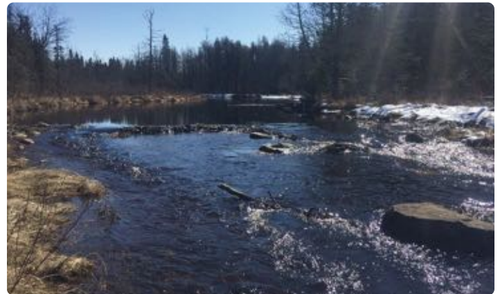
Rock weir at the outlet of Big Rice Lake in 2016. Credit: MN DNR, 2019.
