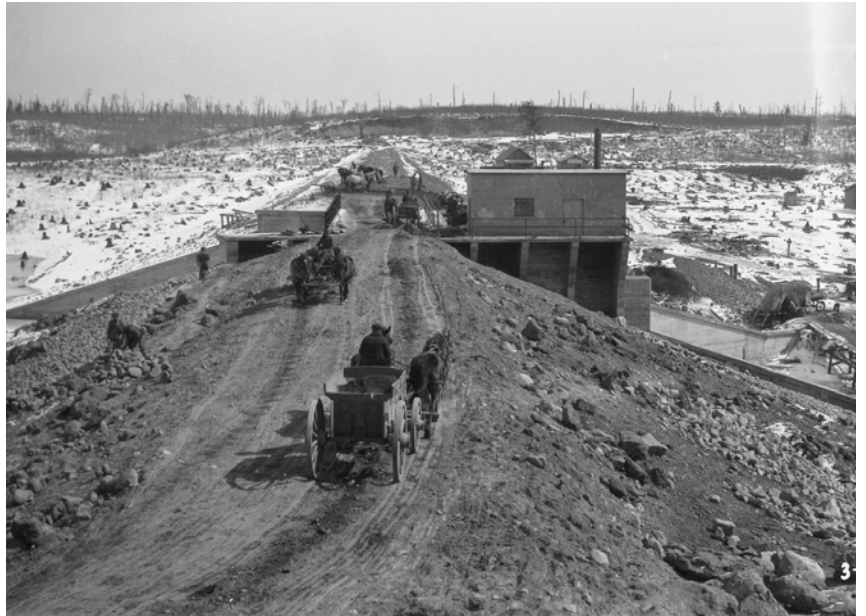
Figure 23. Construction of the Chippewa Flowage.
